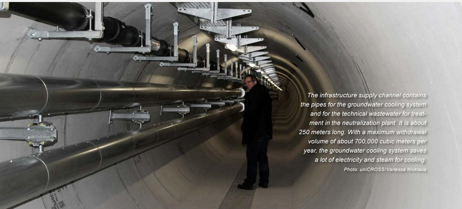
The infrastructure supply channel contains the pipes for the groundwater cooling system and for the technical wastewater for treatment in the neutralization plant. It is about 250 meters long. With a maximum withdrawal volume of about 700,000 cubic meters per year, the groundwater cooling system saves a lot of electricity and steam for cooling.
